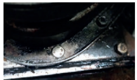
6. The tightened bolt prevents leakage.
